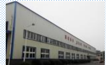
Chongqing Altech New Materials Co., Ltd.
